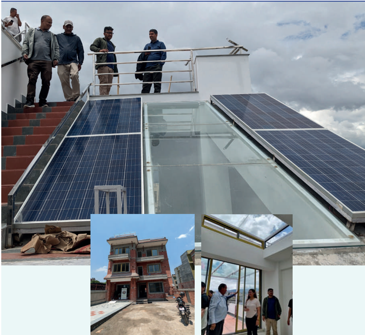
Photo 1: Residential Sector Case Study, Courtesy: Ar. Dibya Acharya, BEEN Project funded by EU under Switch Asia Program
